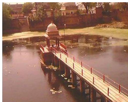
Fig 9: The Water body Surajkund in Fort of Gwalior
