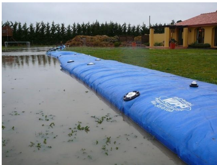
Figure 3: Flood prevention products to replace sand bags
