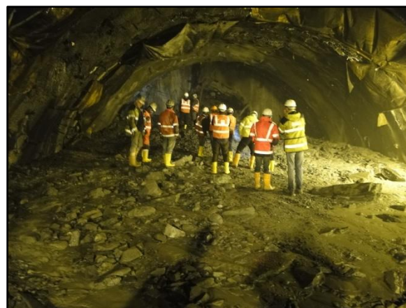
Atal Tunnel under construction
