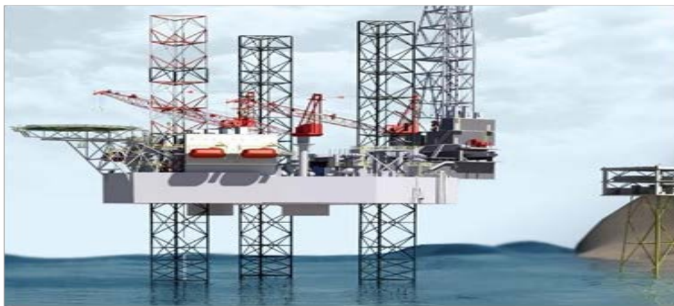
Fig.9 Jack-ups in the elevated positions
