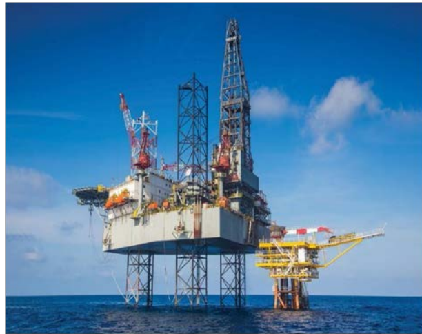
Fig 4 Offshore Telecommunication Towers
