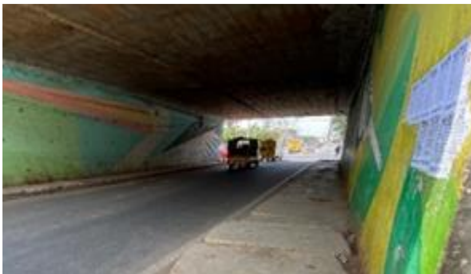
Fig 3: carriage width at underpass
