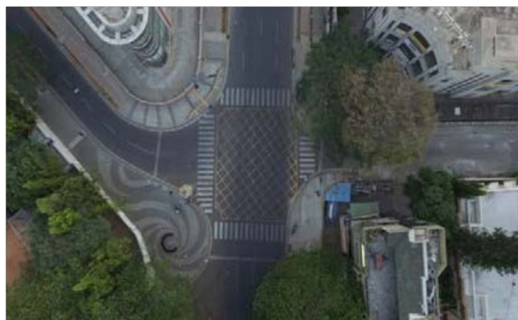
Fig. 4: Tender SURE infrastructure at Richmond road, Bengaluru
