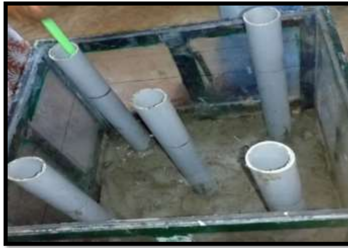
Fig 2 Lime column installation
