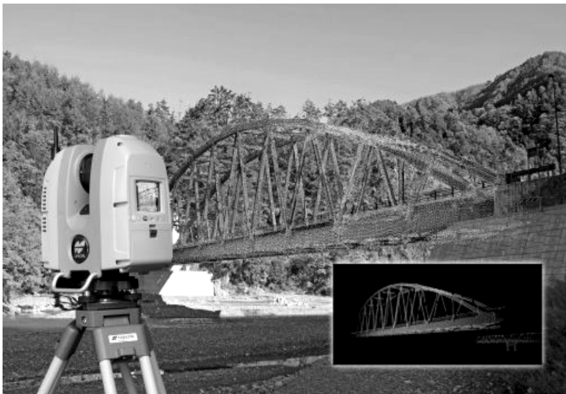
Figure 2 High Definition Scanning to collect point cloud data of a bridge
