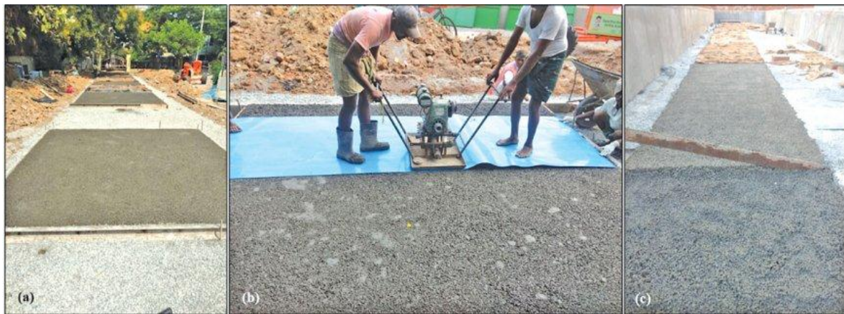
Figure: 4 Construction of pervious concrete pavements
