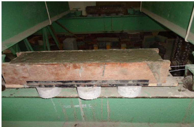
Fig:3 Concreted Prestressed beam
