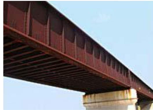
Fig.2: Usage of plate girder in bridges
