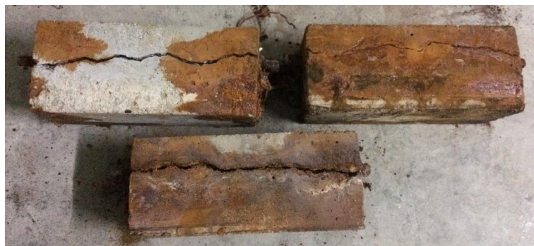
Figure 4: Pattern of Crack
