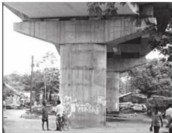
Figure 1 – A Bridge Pier
