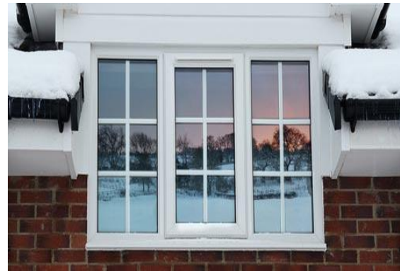
Figure 7: Double pane windows
