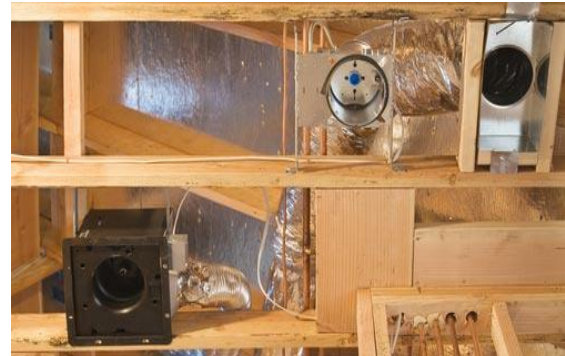
Figure 5: HVAC vents
